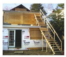
To minimize wear and tear to the finished portion of the house, the crew built a temporary staircase that provided easy access to the third floor from the back yard.
